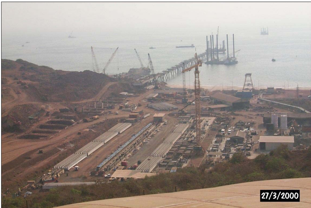
Fig. 9 Precast Yard and Trestle Erection
